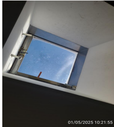
Photo 10 – Overview of the Automatic Opening Ventilation (AOV) unit at the top of the staircase.
