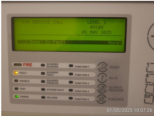
Photo 3 – Fire alarm panel, with error displayed for Zone1
