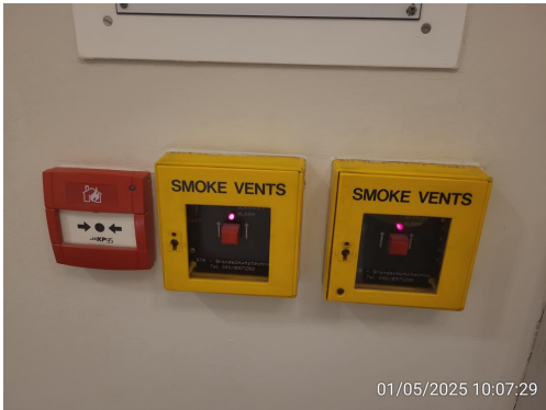
Photo 4 – Smoke vents triggers
