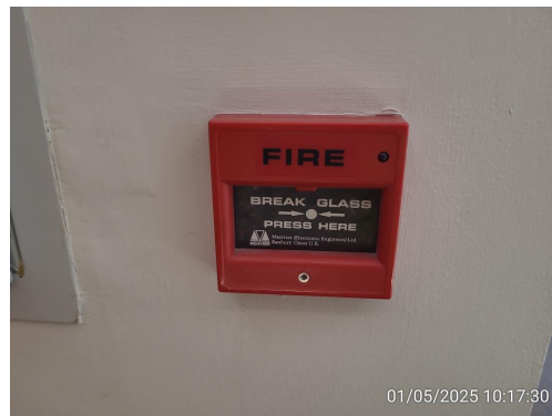
Photo 12 – Fire Alarm call point overview
