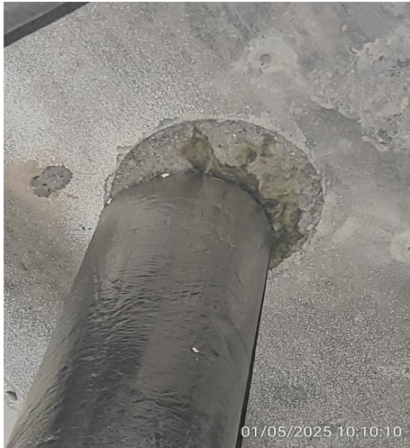
Photo 9 – Some internal compartmentation is carried out with concrete infills
